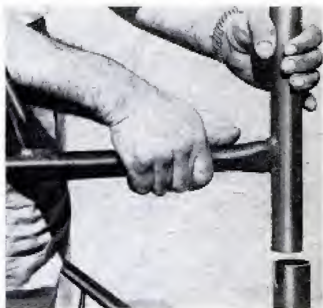
Above, 24-pound frame is basic unit of scaffolding. They slip into each other, below, to form tower, left
